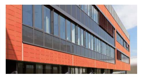
The MB-SE75 system gives architects a wide selection of styles to create individual and stimulating building walls. It is capable of being used in any new construction project from two floors upward. The system is available in regular and advanced thermal insulation varieties. The latter uses special EPDM inserts to increase its insulating properties.
