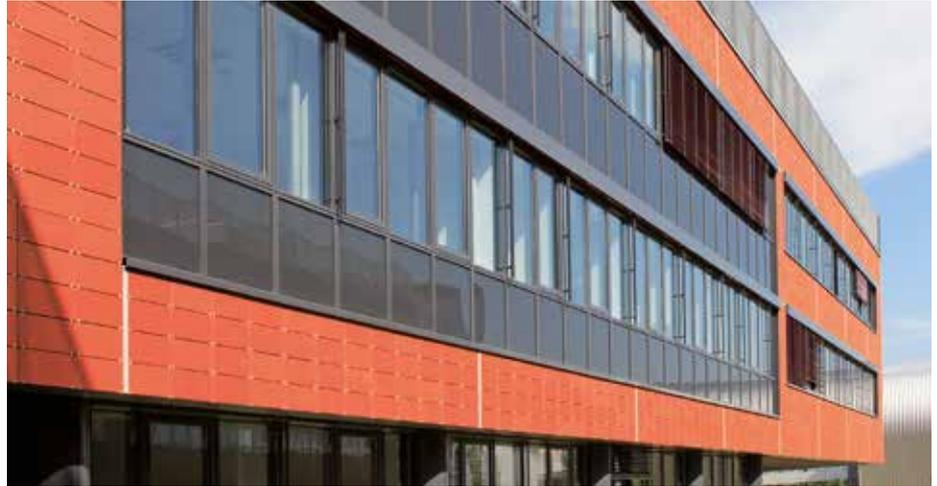
The MB-SE75 system gives architects a wide selection of styles to create individual and stimulating building walls. It is capable of being used in any new construction project from two floors upward. The system is available in regular and advanced thermal insulation varieties. The latter uses special EPDM inserts to increase its insulating properties.
